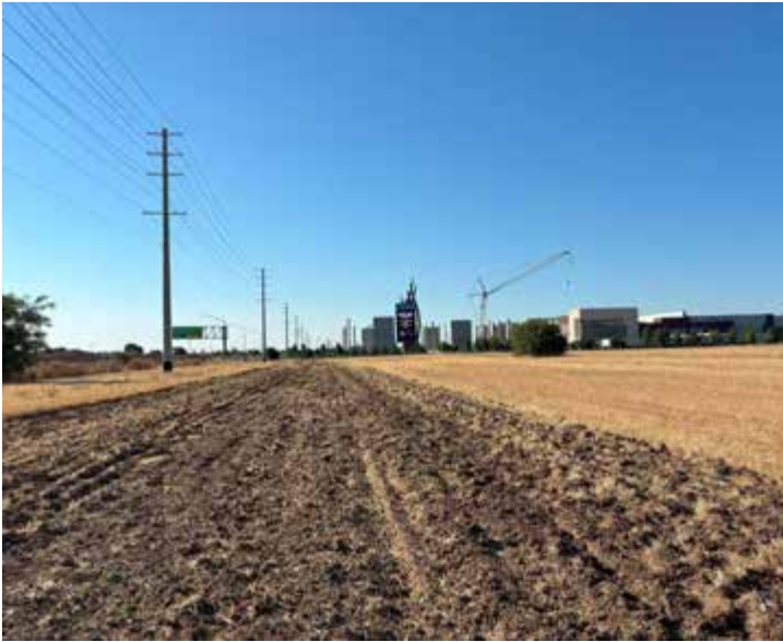
View of the northernmost parcel facing the Sky River Casino to the south.
