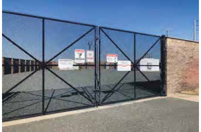
SMUD Substation north of Subject Property.
