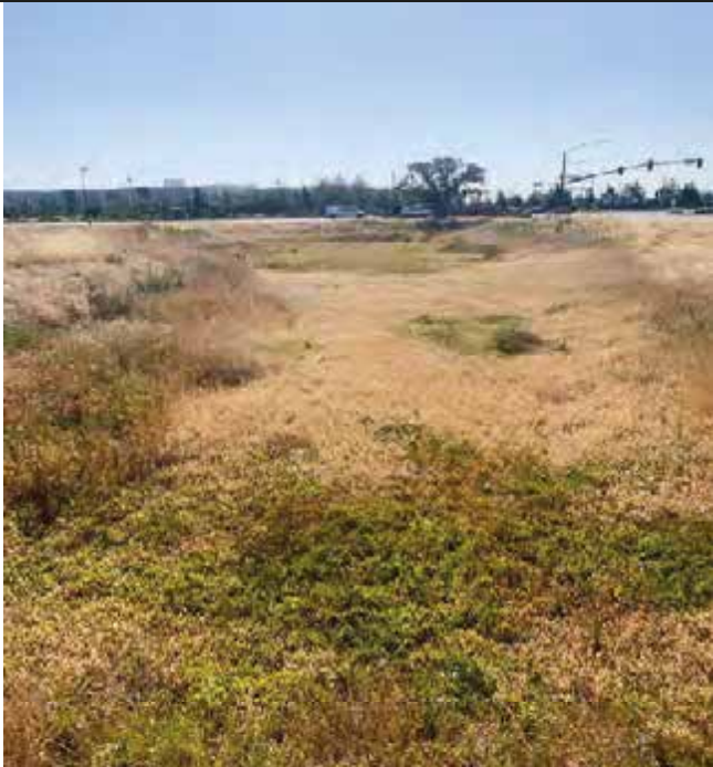
Stormwater Basin in APN 134-1010-0005. Looking east
