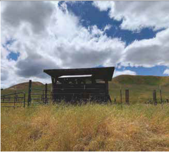
Historic ranching structure adjacent to the corral in the northeaster corner of the Subject Property.
